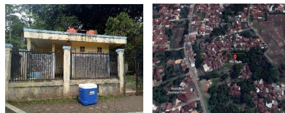
Figure 3. Building Sanimas Cipaku Village, Paseh District
