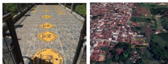
Figure 1. Building Sanimas Neglasari Village, Banjaran District
