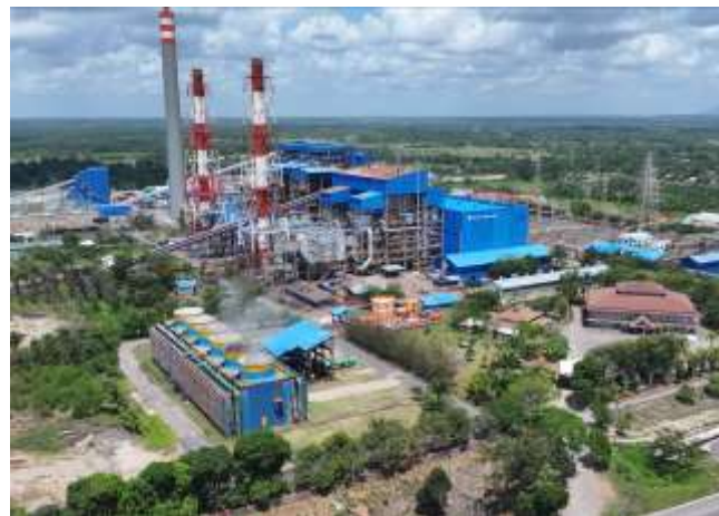
Figure 1 Asam Asam Coal-Fired Power Plant
