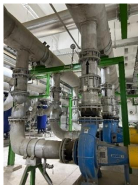
Figure 2. Centrifugal Pump
