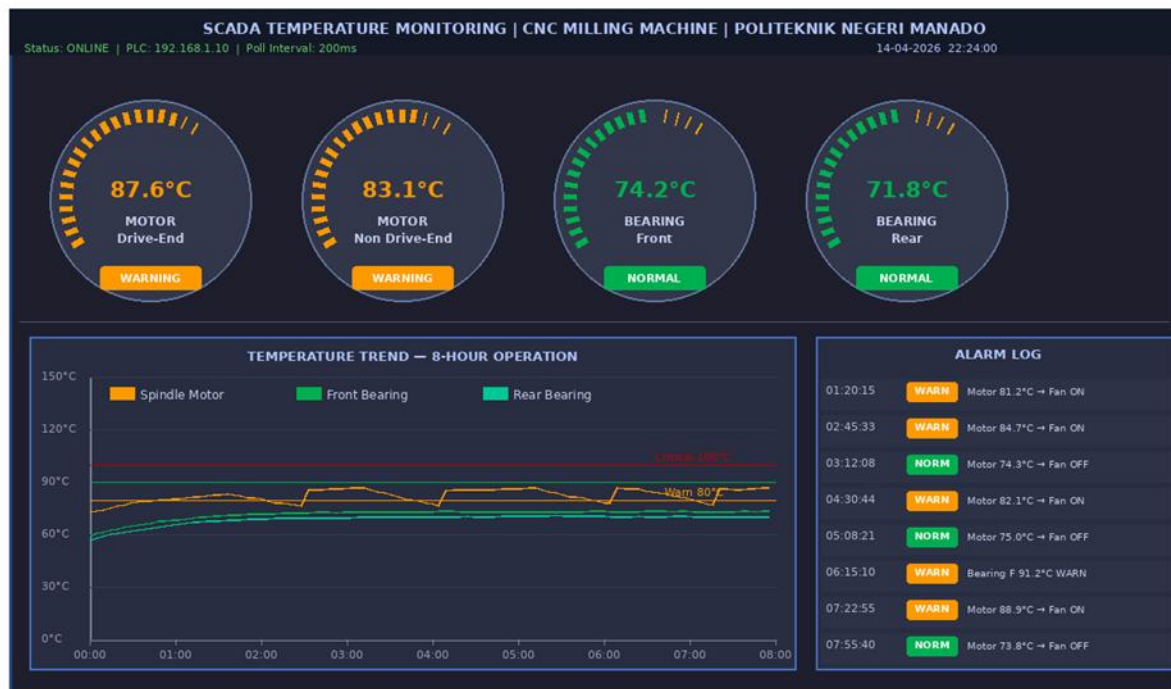
Figure 4. SCADA HMI main screen displaying real-time temperature gauges, 8-hour trend chart of spindle motor and bearing temperatures, and alarm event log during full-load operation.
