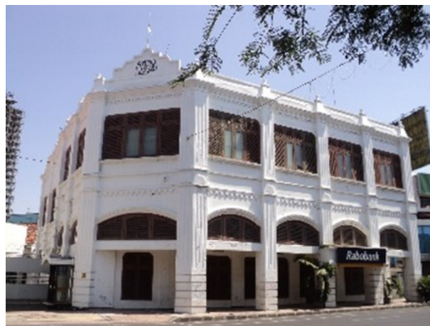
Image 1. Hagakita Bank Building
