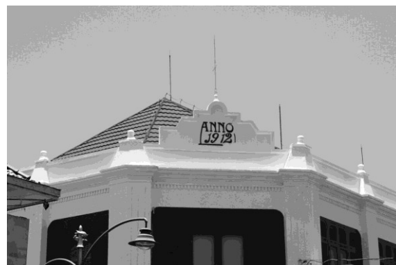
Image 3. Roof of Bank Hagakita Building Source: Pinterest, 2025
