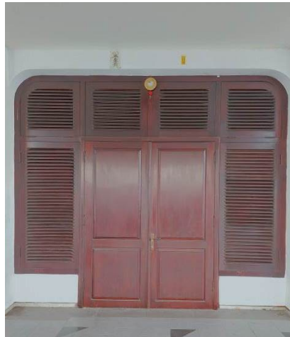
Image 4. Bank Hagakita Building Window Source: Researcher, 2024
