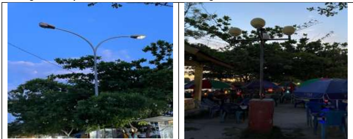
Figure 18 Condition of Park Lighting (Source: Personal Documentation)
