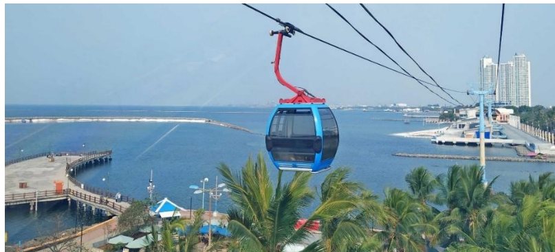
Fig. 2 Ancol Gondola Cable Car (Source: Gondola-Ancol.com)
