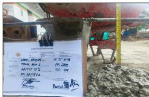
Figure 7. Slump Test on 5% mixture Sikacrete-W
