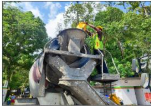
Figure 5. Additive Pouring
