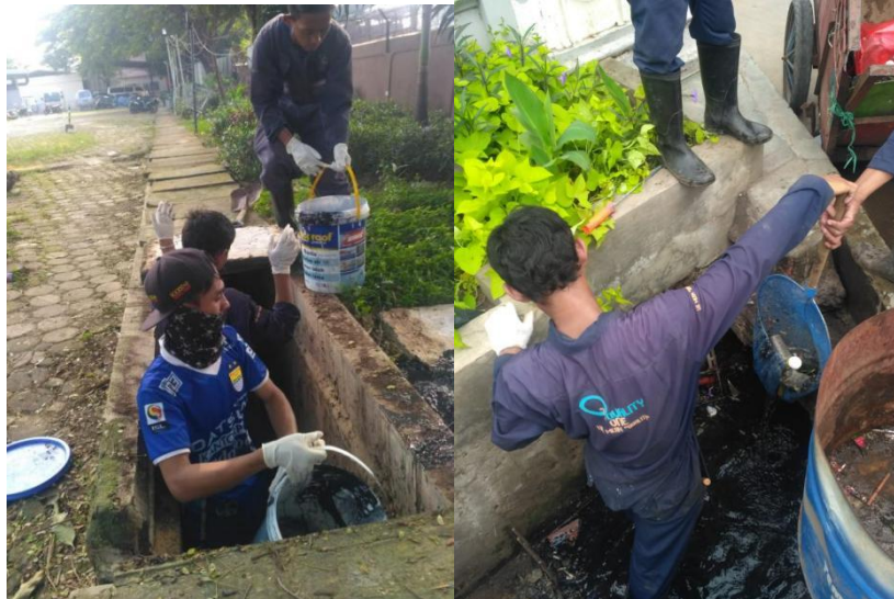
Figure 1. Image Cleaning and treatment of wastewater lines at Hospital X
