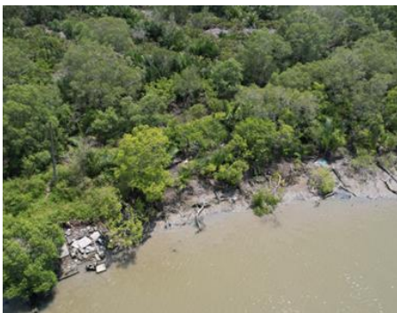
Figure 1. Critical Cliff Location
