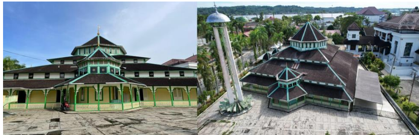
Figure 14. Building shape (Source: Author, 2023)
