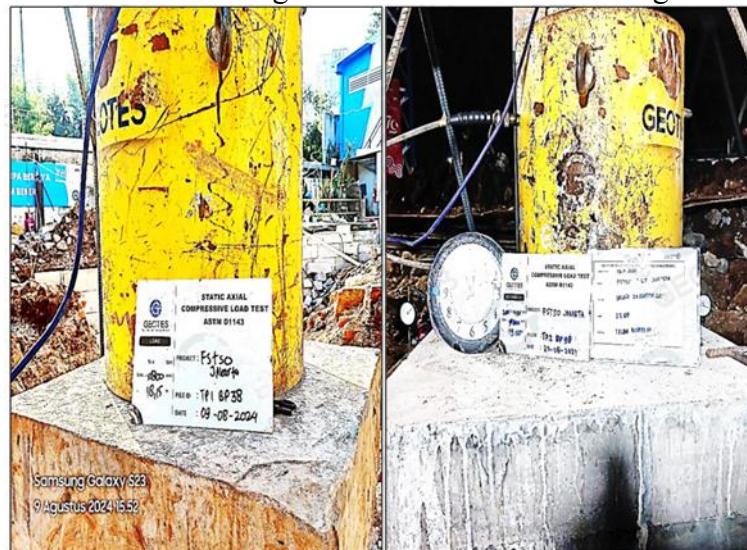
Figure 4. Documentation of Axial Testing of Pile Foundations
